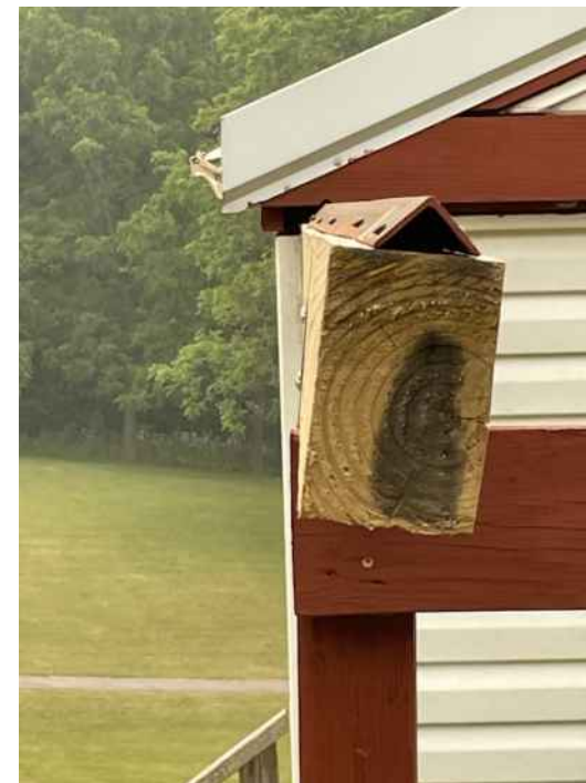
This rail on the Brew House was repaired in 2023
